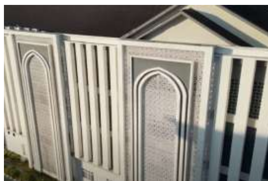
Figure 11: Ventilation Panels on facade
